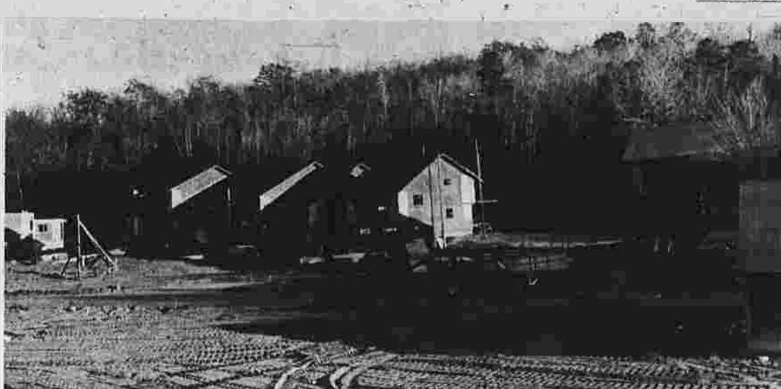
Development taking shape First Hartford Realty Corp.'s Forest Ridge 60-unit project has been designed as a luxury Condominiums are under construction on a 28.7-acre site off Lydall St. and Greenwood Dr. The complex, starting prices are expected to be in the $50,000 to $80,000 range.
